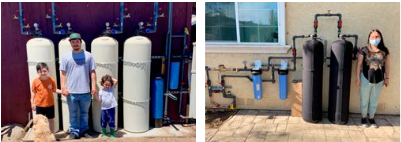
Figure 1: Project participants in front of a 24-cubic foot system (DWMC-09) near Salinas (left), and a CWC staff member next to a 7.2-cubic foot system, DWMC-19 in Royal Oaks (right).
