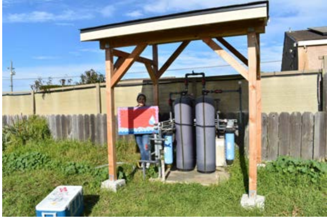
Community partner María Gonzalez next to DWMC01 with installed shade structure.
