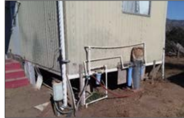
Phase 2B Installation Site
