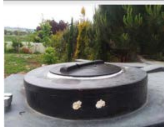
New tank lid installed
